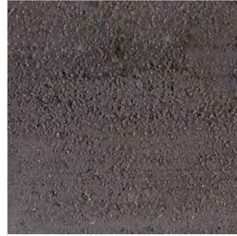
Primary / Secondary Path - Coloured concrete
