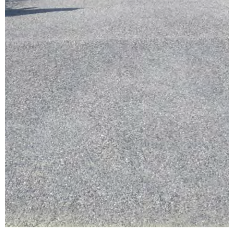
Primary Path - Exposed aggregate concrete
