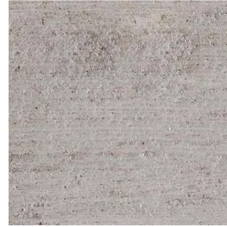
Primary / Secondary Path - Coloured concrete
