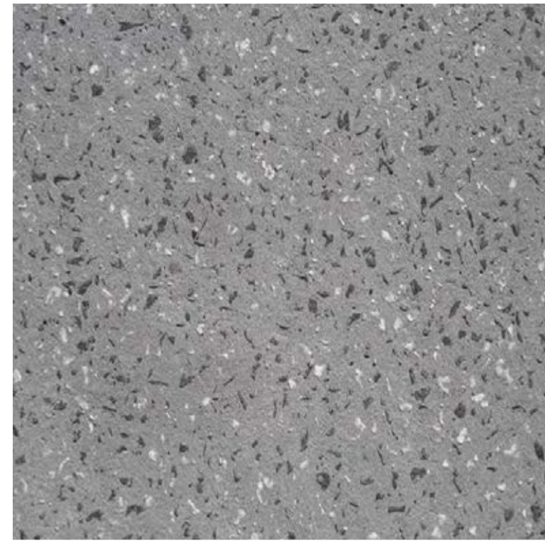
Primary Path - Exposed aggregate concrete
